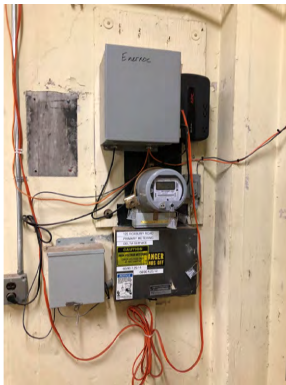
Figure E-16 Primary Electric Service Metering in Building 3
