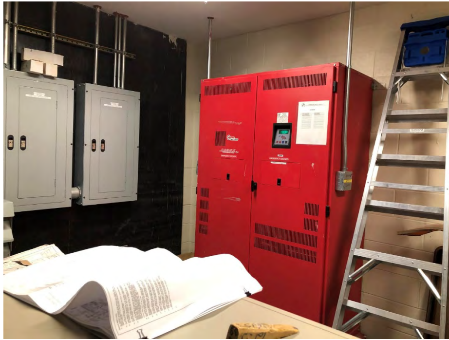
Figure E-12 Central Emergency Lighting Inverter System and Electrical Distribution System in Building 1
