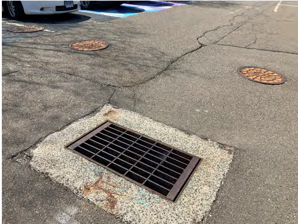
Photo 13: Typical Catch Basin and Storm Drainage Manholes
