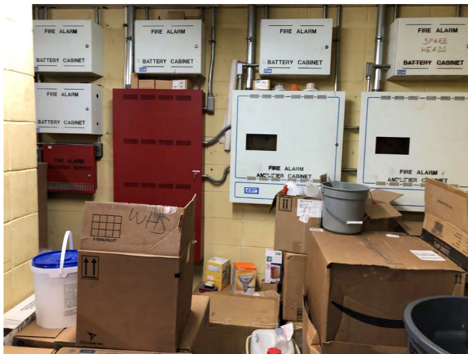
Figure E-18B Associated Booster Panels and Battery Cabinets for Fire Alarm System in Building 3
