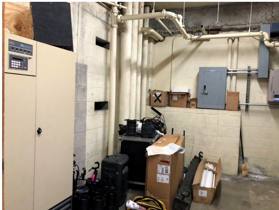
Figure E-19 Emergency Lighting Inverter in Storage Room Adjacent to Stage in Building 3
