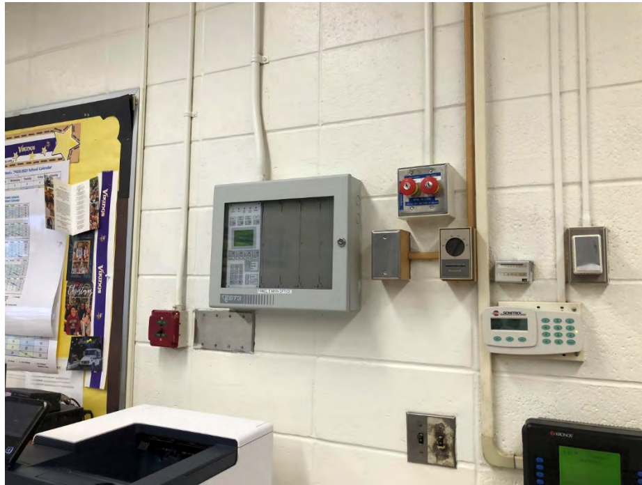
Figure E-18C Remote Fire Alarm System Annunciator Panel Located in Administration Office in Building 3
