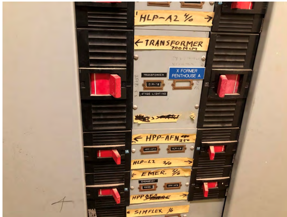
Figure E-15A Distribution Section of Main Switchboard MDB1 Located in Switchgear Room in Basement under Stage in Building 3
