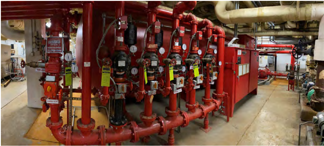
Figure E-17 Fire Pump and Fire Pump Controller in Building 3
