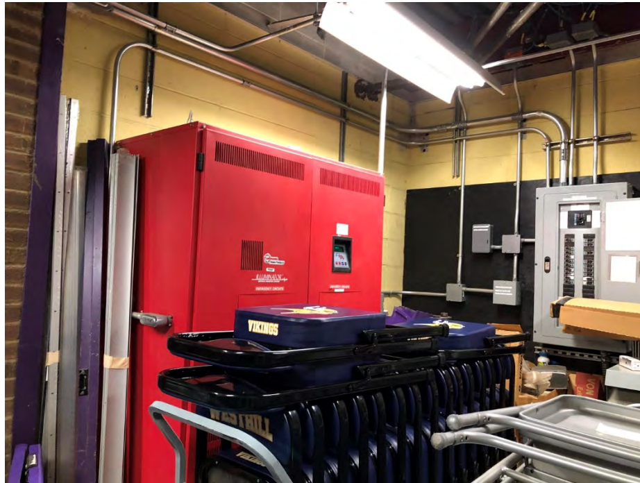
Figure E-9 Central Emergency Lighting Inverter System and Electrical Distribution System for Building 2 Located in Building 2A
