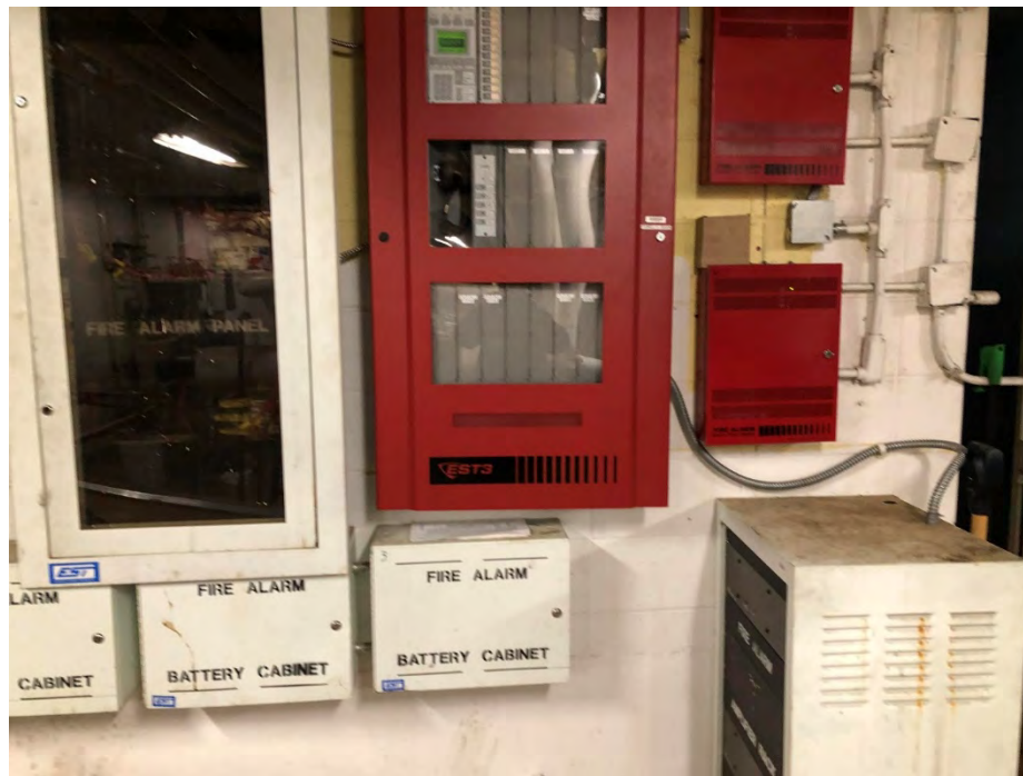
Figure E-18 Main Fire Alarm Control Panel and Associated Equipment in Building 3
