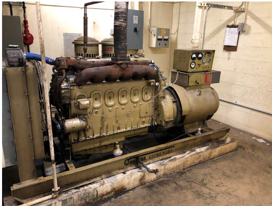
Figure E-14 125 kVA / 100 kW Interior Building-Mounted Generator for Emergency Lighting in Building 3
