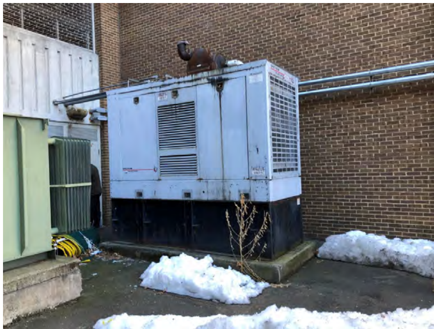
Figure E-2 Site-Mounted Generator Serving Fire Pump Located in Mechanical Room on Lower Level of Building 3
