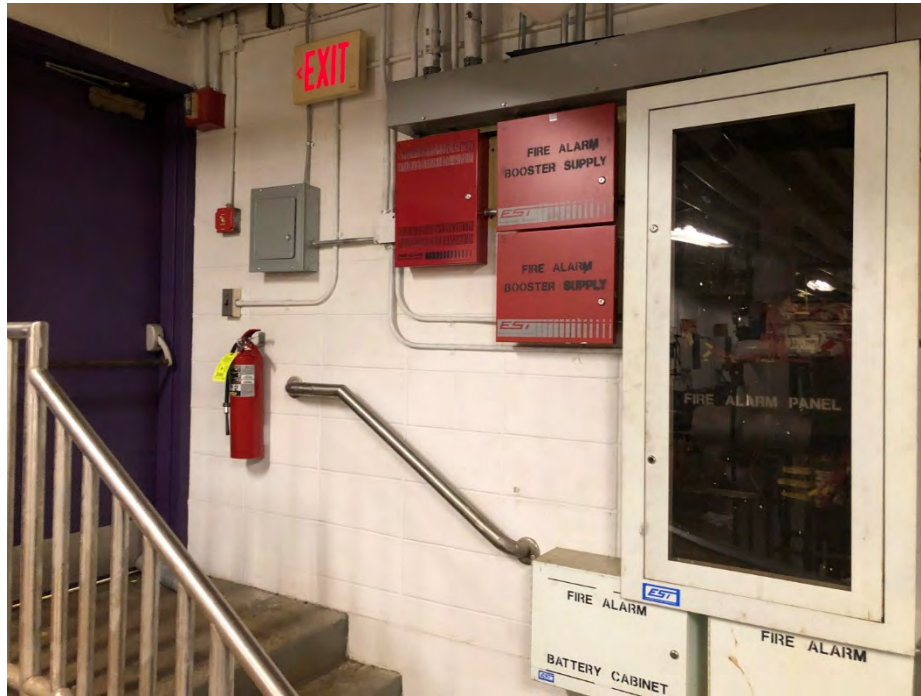
Figure E-18A Main Fire alarm Control Panel and Associated Equipment in Building 3
