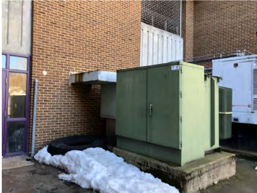
Figure E-1 Site-Mounted Utility Transformer Serving Main Switchboard MDB2
