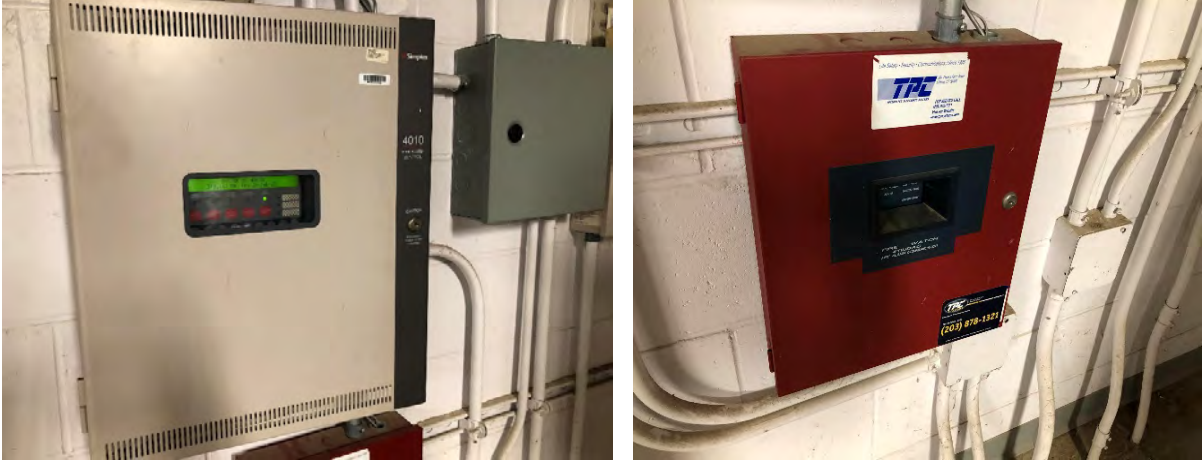
Figure E-24 Fire Alarm System Control Panel with Fire Alarm Communicator in Building 5
