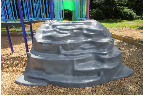
Toad Stool Climber (1) - Loose at post - MAINTENANCE
