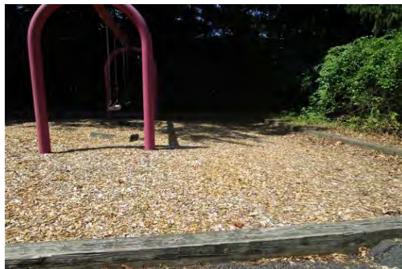
7ft. Swing Set (1Bay/2Belts)(GT) - Surfacing, low towards back - MAINTENANCE
