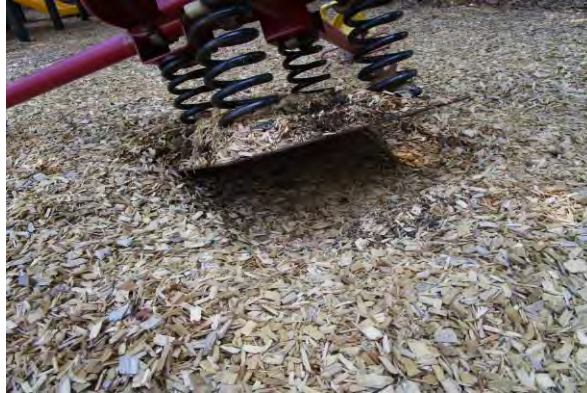
Structural Stability - Not anchored - CLASS B HAZARD
