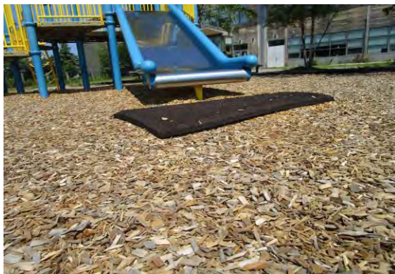
Surfacing - Non-beveled wear mat not level, tripping hazard - CLASS B HAZARD
