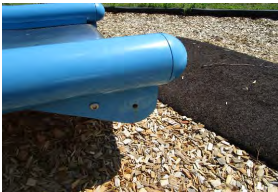
Wide Toboggan Slide (metal) - Two bolts missing at bottom of bed way - MAINTENANCE
