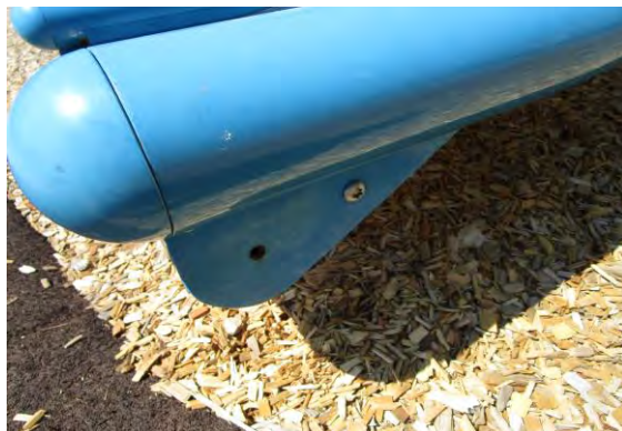
Wide Toboggan Slide (metal) - Two bolts missing at bottom of bed way - MAINTENANCE
