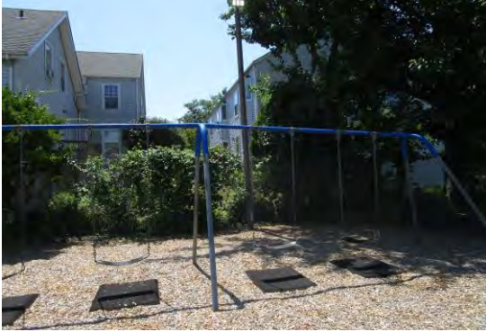
9ft. Swing Set #2 2Bay/4Belts) - Four belts seats wearing - MAINTENANCE
