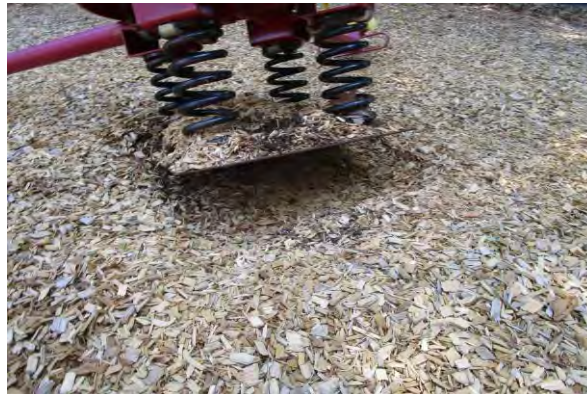
Structural Stability - Not anchored - CLASS B HAZARD
