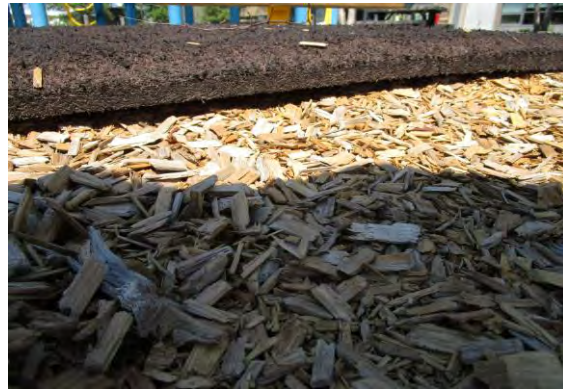
Surfacing - Non-beveled wear mat not level, tripping hazard - CLASS B HAZARD
